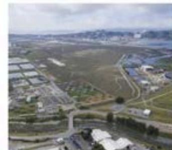
10 West County Wastewater Facility
